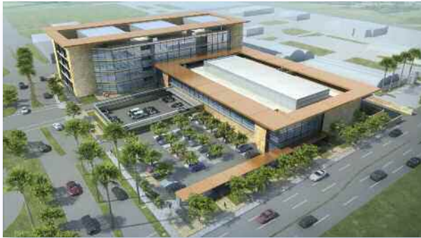
East County Detention Center Off-Site Improvements
