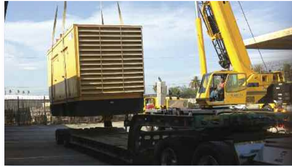
Power generator upgrade
