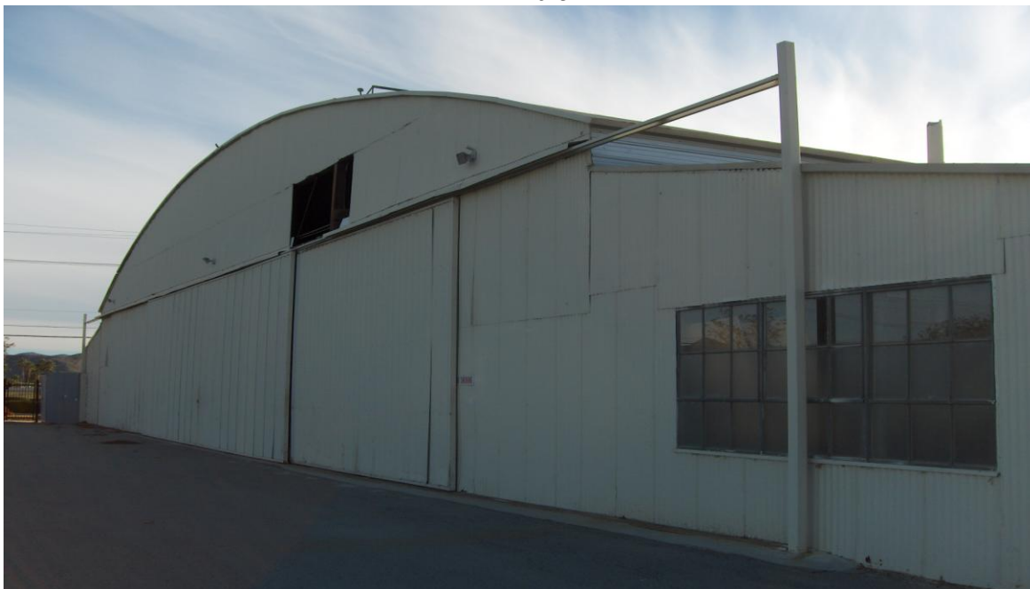
Figure 2: Hemet Ryan Hangar #4Demolition
