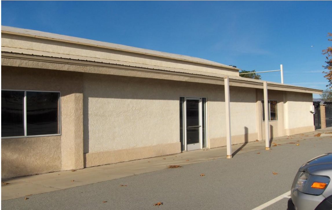
Figure 1: Hemet Ryan Hangar #4Demolition
